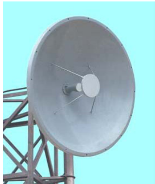
Figure2.4 Parabolic antenna
