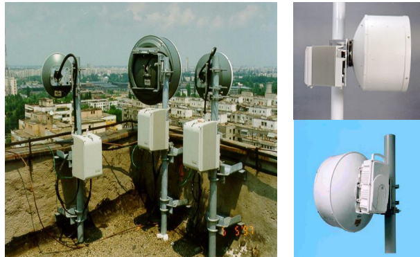
Figure 2.8 Antenna connected to ODU
